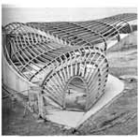
3.55a-c. Use of ruled surfaces in the Water Pavilion (1998), the Netherlands, architect Lars Spuybroek/NOX Architects.
