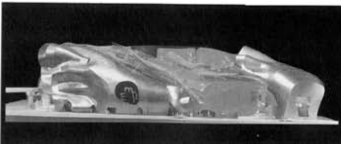
3.9a-b. Experience Music Project (EMP) (2000), Seattle, USA, architect Frank Gehry: 21,000 differently shaped metal shingles for the exterior were cut digitally.
