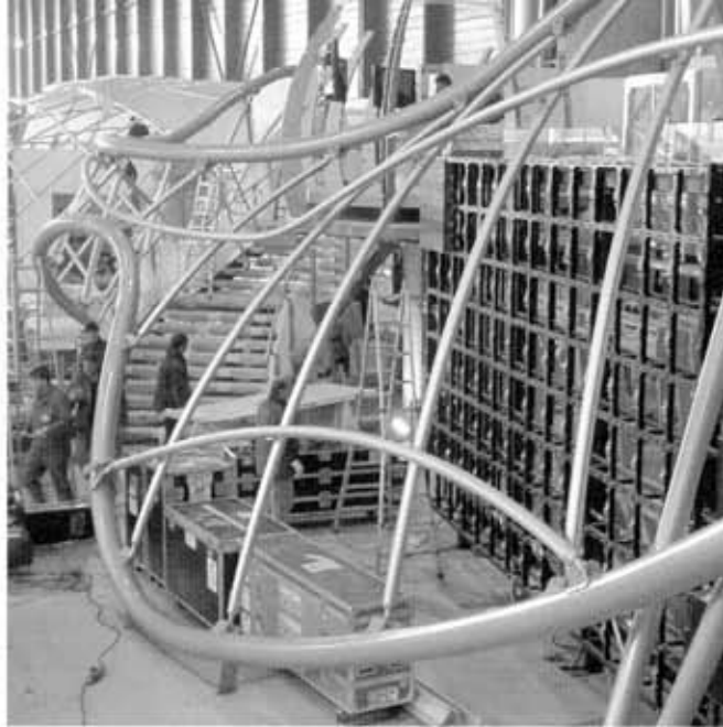
3.40. Assembly of the "Brandscape" BMW Pavilion at the 2000 Auto Show in Geneva, Switzerland, architects Bernhard Franken and ABB Architekten.
