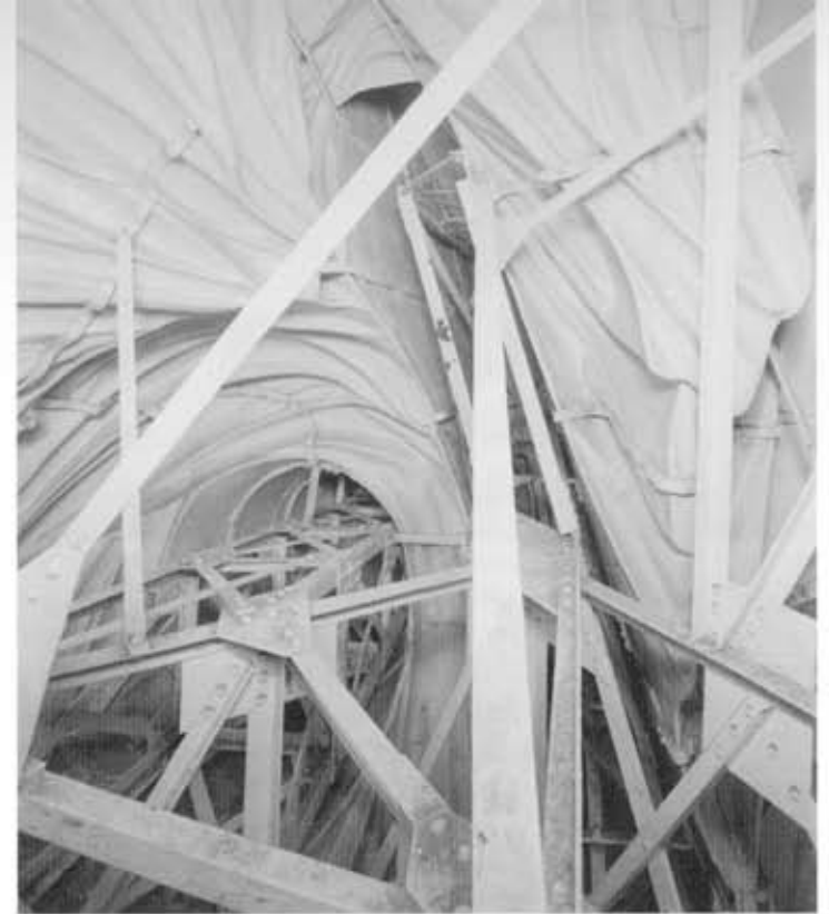
3.35. Statue of Liberty (1886), New York, architects Gustave Eiffel and Auguste Bartholdi: folds, armature and bracing.
