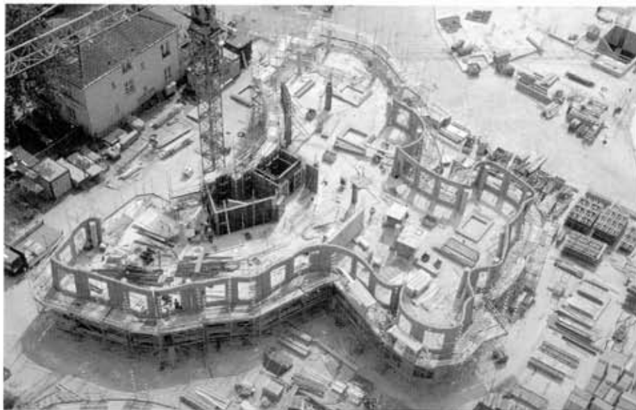
3.17a–f. The reinforced concrete panels for Gehry's Zollhof Towers (2000) in Düsseldorf, Germany, were precast in CNC-milled Styrofoam molds.
