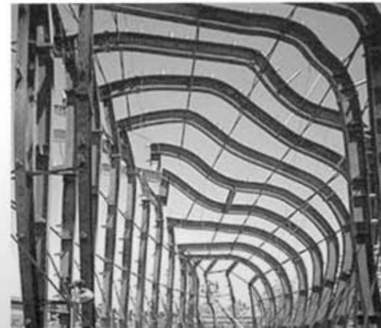
3.35. Statue of Liberty (1886), New York, architects Gustave Eiffel and Auguste Bartholdi: folds, armature and bracing.
