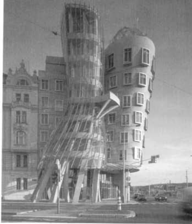
3.8a-b. Nationale-Nederlanden Building (1996), Prague, Czech Republic, architect Frank Gehry: irregularly-shaped glass panels were cut using digitally-driven cutting machines.
